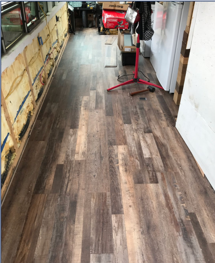
New temperature-resistant flooring with a bamboo core to negate expansion and contraction.
