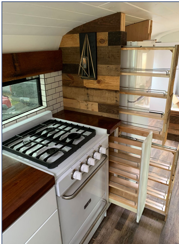
Rev-A-Shelf soft close pullouts installed in the kitchen.
