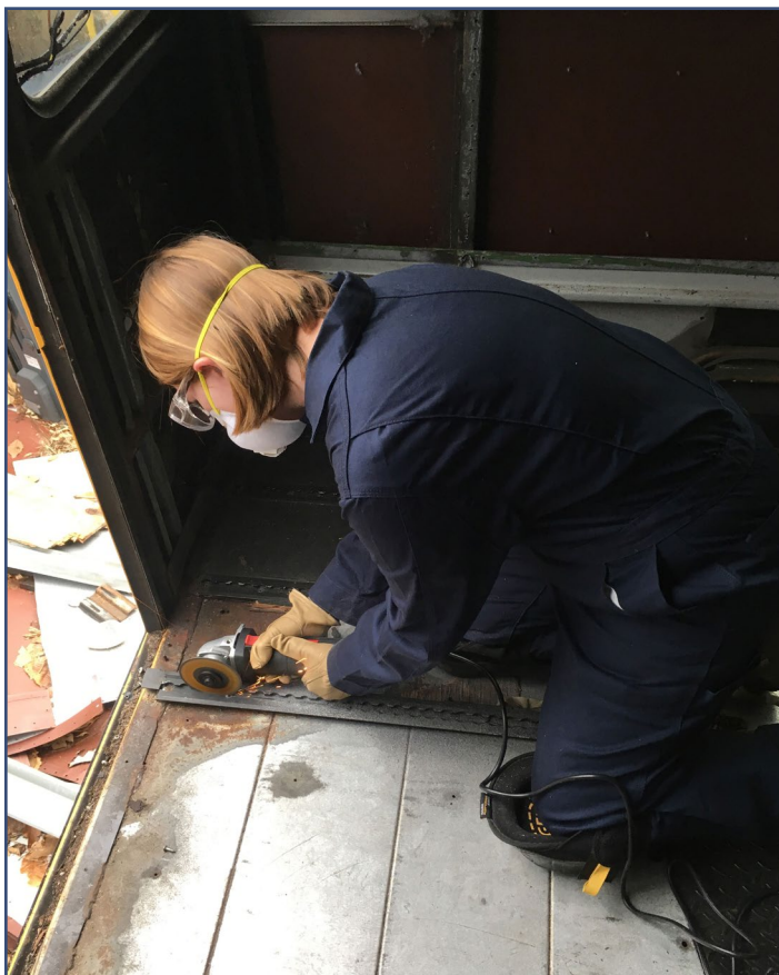
Cutting out the L-tracks.
