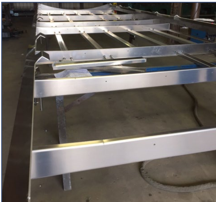
Solar rack fabrication in full swing.
