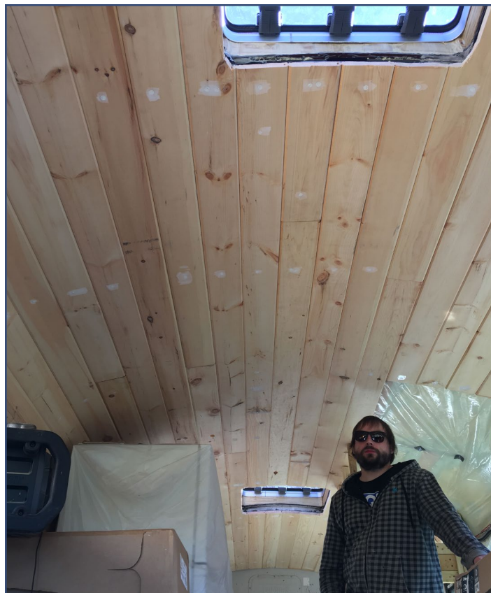
Reinstalled, unpainted ceiling.
