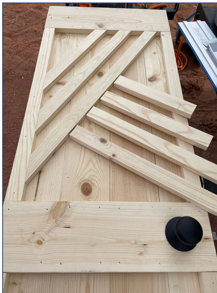
Constructing the bathroom door.
