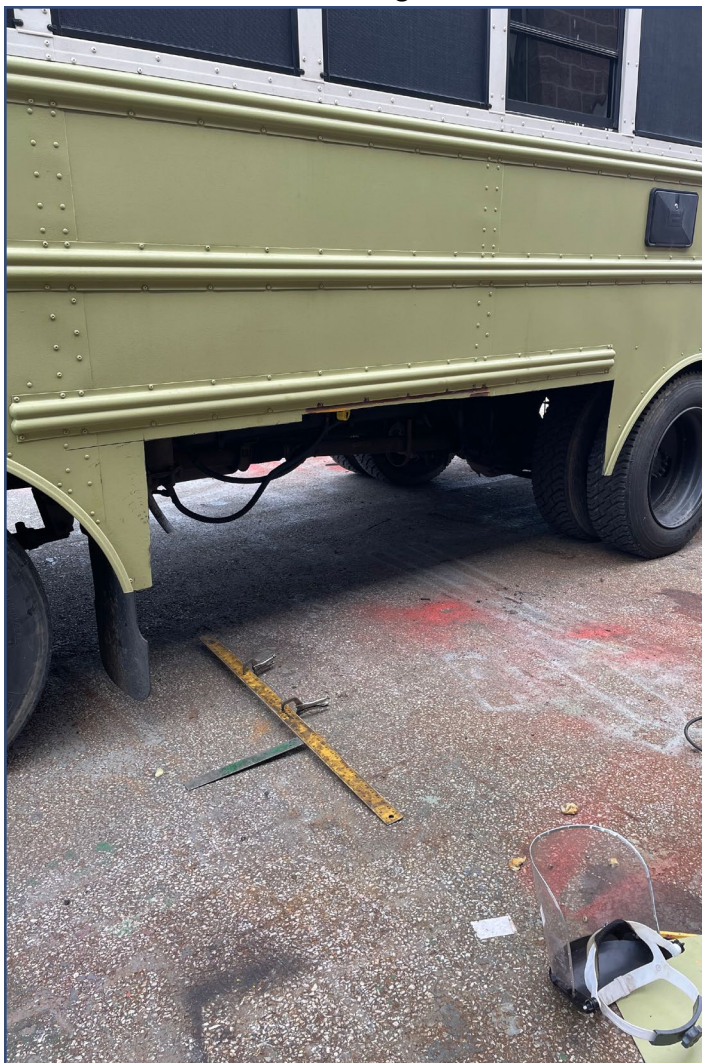
Cutting the sheet metal in preparation for the toolbox installation in the middle of the bus.
